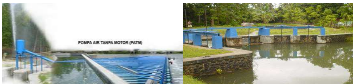
Pompa Air Tanpa Motor/PATM
